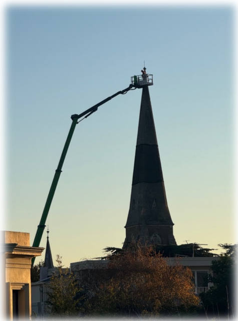
Adding safety nets to the spire
