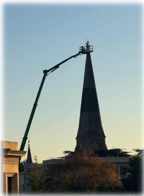
Adding safety nets to the spire
